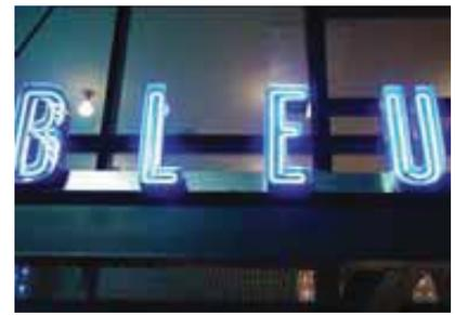
Open pan channel letterforms with recessed exposed neon.
